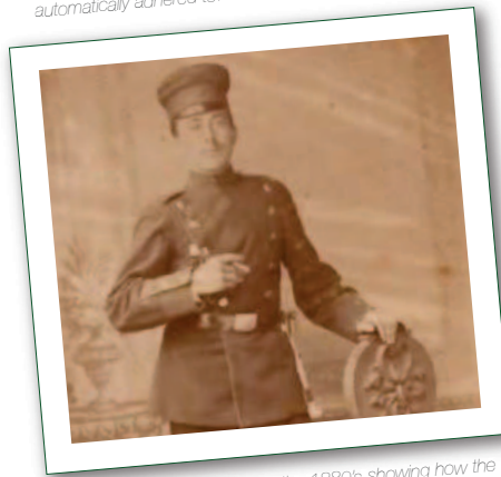
An earlier photograph dating from the 1880's showing how the service cap's height gradually extended during this period.
